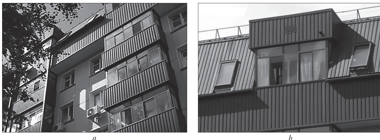
Fig. 6. Pilot project of residential house reconstruction without resettlement of inhabitants in Kharkiv (Ukraine): a — building's façade; b — added mansard
