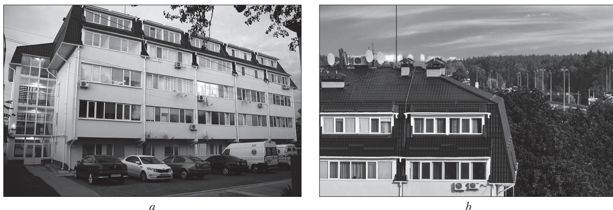
Fig. 1. Reconstruction of low-storey large-panel houses in the city of Erfurt (Germany): a — an added mansard; b — upper-floor balcony conversion into loggia
